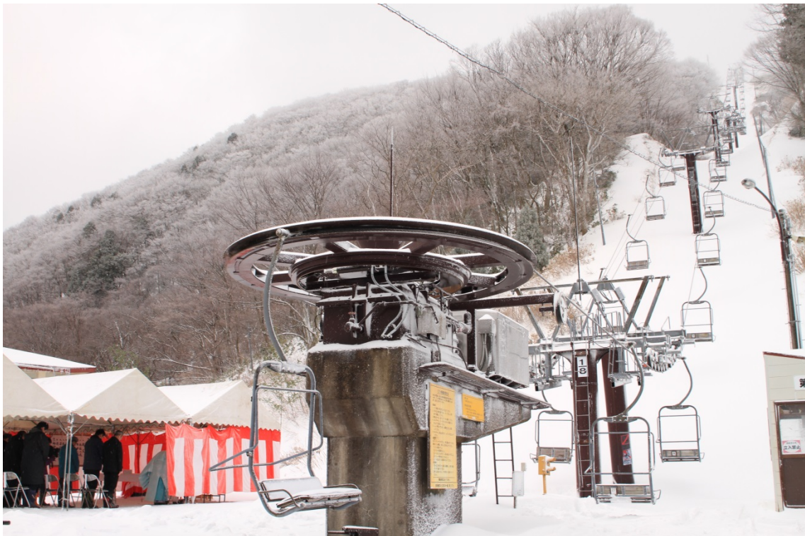
↑ After the Safety Prayer Festival, the first lift underwent a test run.
