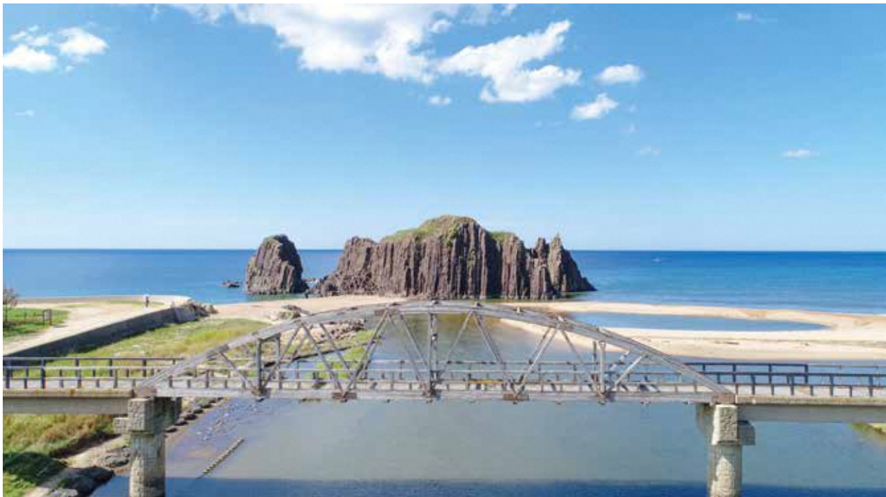
京丹後市の中央部を流れる竹野川を正面で受け止める立岩 The view of Tateiwa Rock from the Takano River, which runs through the center of Kyotango
